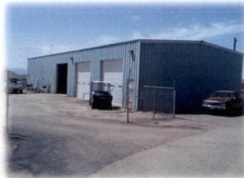
Old Public Works Building built in 1972
